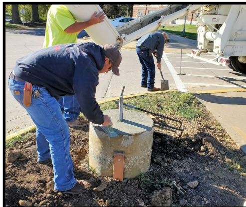
New light pole base
