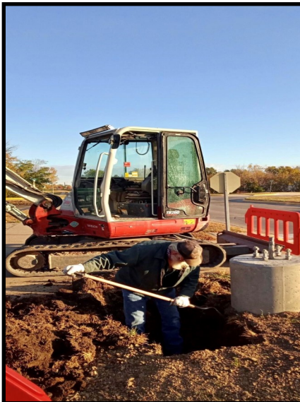
Running underground electrical wires
